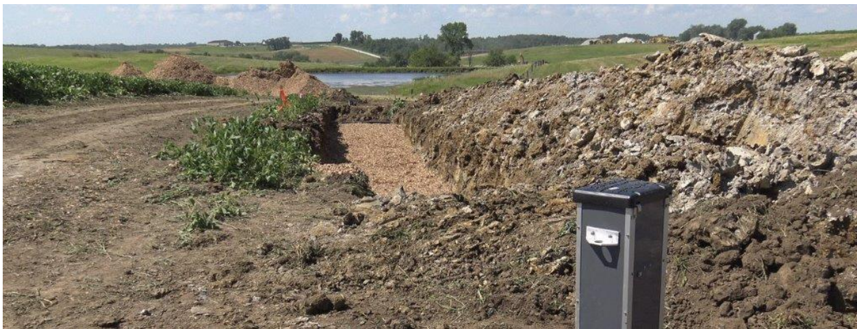
Figure 7.4. The construction of a bioreactor. Photo credit: Iowa Soybean Association.
