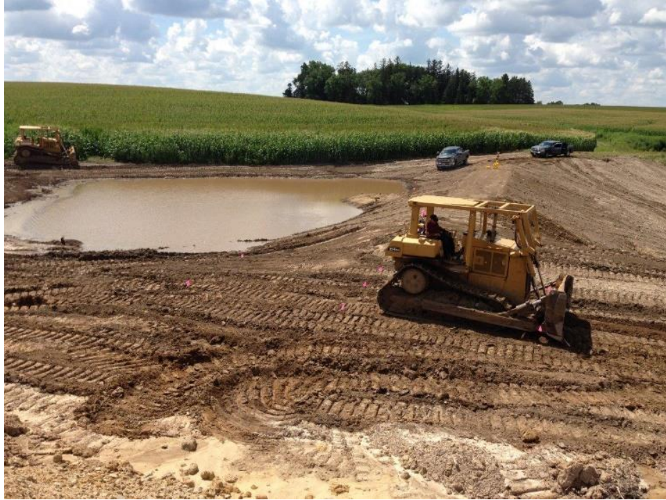
Figure 6.2 A water and sediment control basin under construction. Photo courtesy: Minnesota Department of Agriculture.
