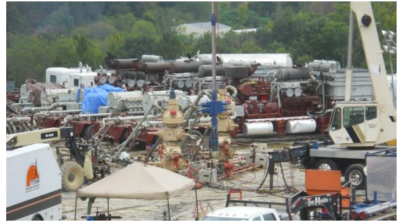
Hydraulic fracturing in progress. Photo credit: USGS.
